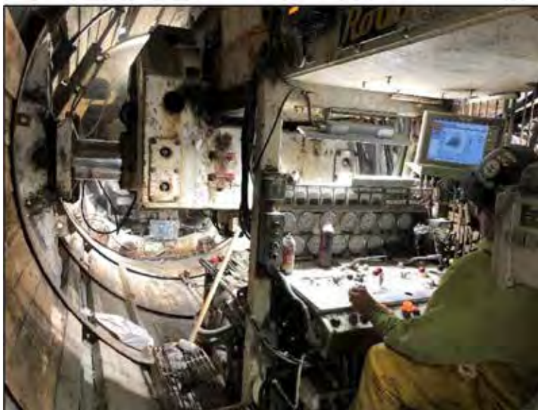
WCT TBM operations.
